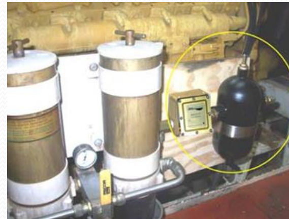
Dieselcraft 5x16 Purifier on Perkins 503 KW Generator in Port Said, Egypt
