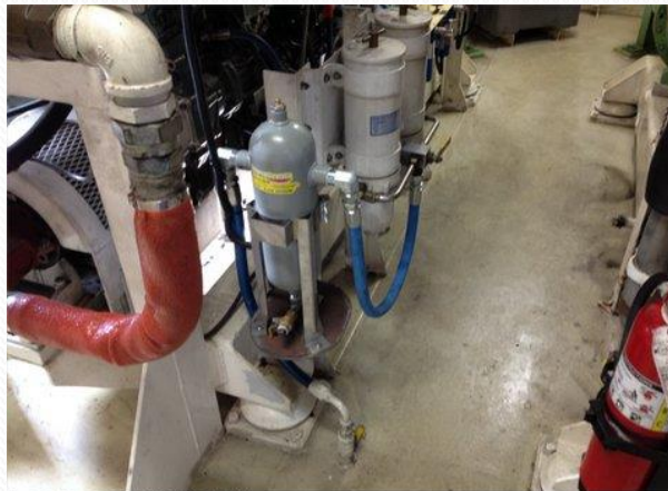
Dieselcraft 5x16 Purifier with stand on 650 hp MTU Engine in fuel barge
